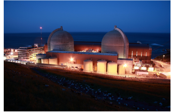
Diablo Canyon in California is among several carbon-free, baseload-producing nuclear power facilities that have closed in recent years.
