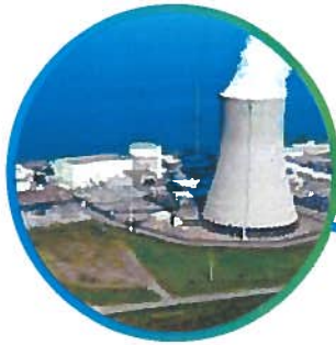
Nine Mile Point Nuclear Generating System
