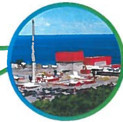
FitzPatrick Nuclear Power Plant
